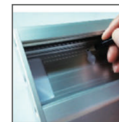
Mark the position of mounting openings
