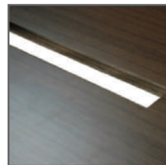
With the dimensions provided in "Recommended Cutout dimensions" prepare recess channel on the table
